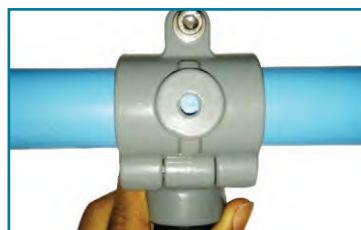
Step 2: Marking the position of the hole on tube
