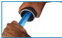
Step 2: Chamfering the Tubes
