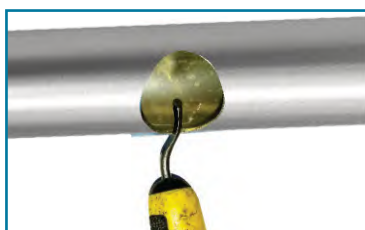
Step 4: Chamfering the hole
