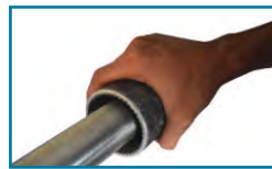
Step 3: Chamfering the Tubes
