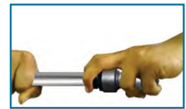
Step 5: Inserting the Tubes into fitting
