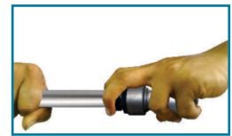
Step 5: Inserting the Tubes into fitting
